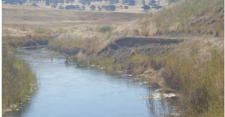
Figure 1 – UFC slide area after repair, June 2016
