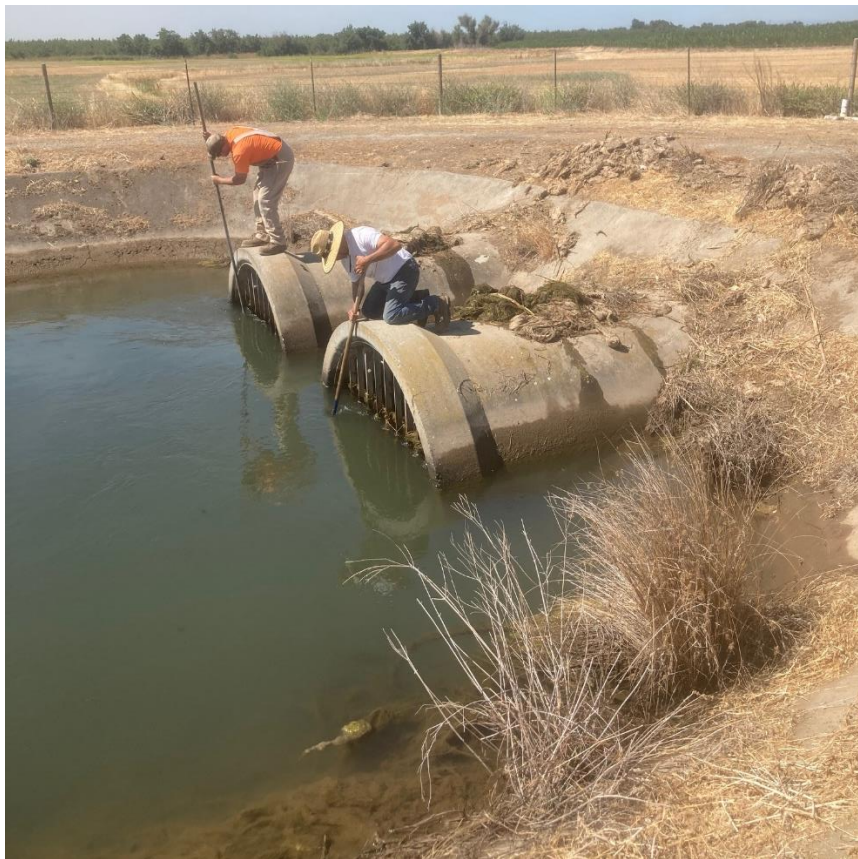
Figure 4. Cleaning Siphon Grates at North Fork of Duck Creek
