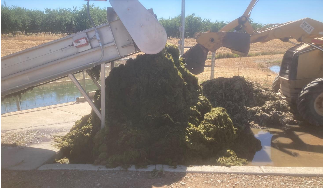
Figure 3. Vegetation Removed at Escalon-Bellota Road Trash Rack
