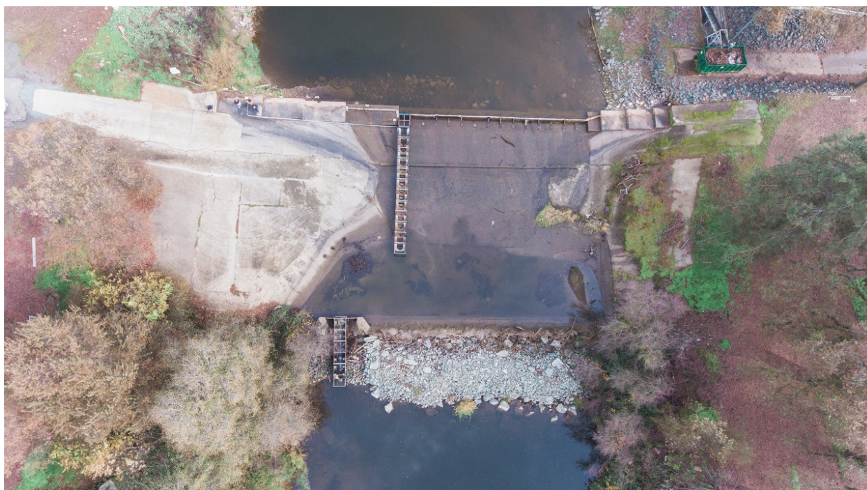
Figure 14. An overhead view of the Bellota Dam and fish ladders under low flow conditions. Note how the lower pool is disconnected from the upper pool preventing fish passage without the assistance of ladders.
