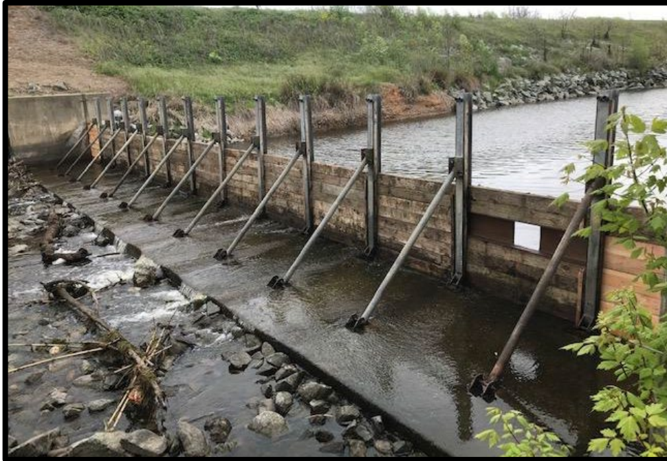
Figure 2. Fish Notch Installation
