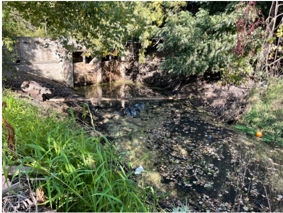
Clements Dam, October 16, 2021
