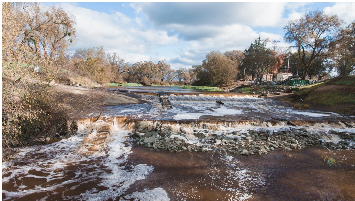
Figure 13. A view of the Bellota Dam structure and the existing two fish ladders looking upstream.
