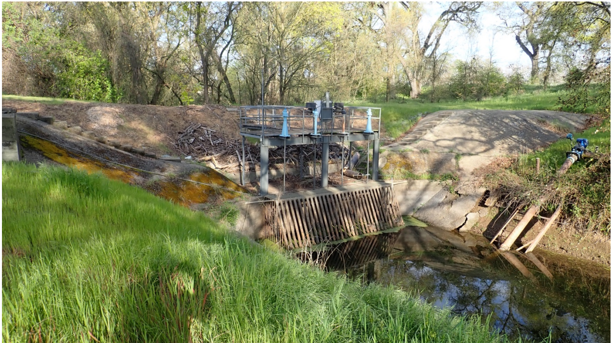
Figure 24. Old Calaveras Headworks structure.
