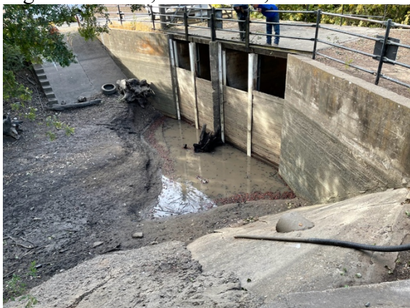
Pezzi Dam, October 13, 2021
