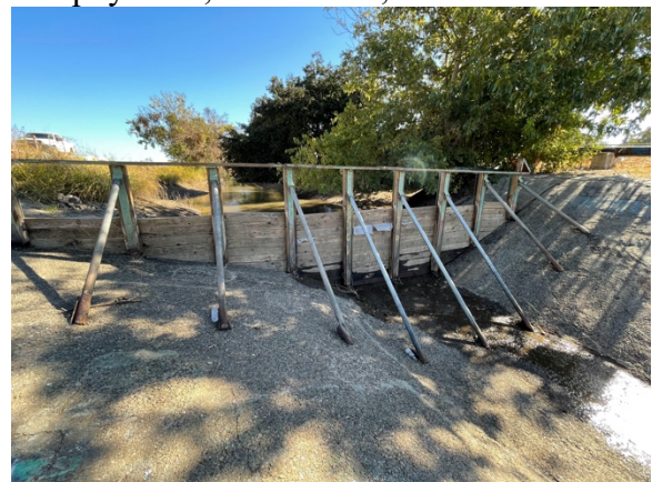
Cherryland Dam, October 14, 2021
